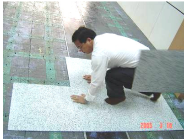
Install Actile on access floor same procedure as PVC tile.
