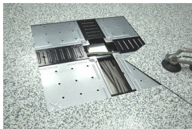
Remove old carpet tiles. Brushing releasable adhesive.
