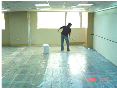
Remove old carpet tiles. Brushing releasable adhesive.
