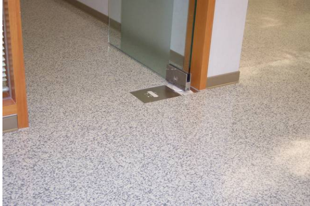
Meeting room door hinge installed on AN45 panel
