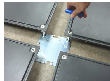
steps 2 adjust height from top by key wrench
