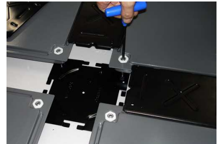
Step 1 and 3: to loose and lock Socket Set Screw from above
