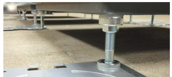
S 4 mm hex key wrench + pedestal at the lock-nut at bottom
