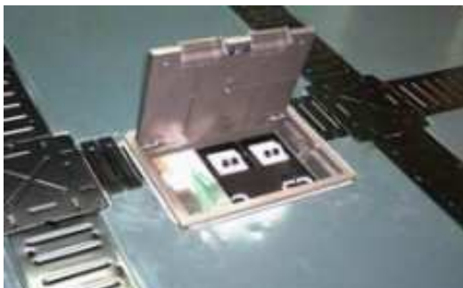
To accommodate large size floor box - Cut at side of the panel (count in the Cable Trench width) and installed at the trench.
