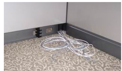
Cables extending from Cable Trenches to wallbase, desktop, any point of the workstation
