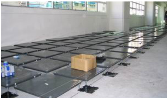
Self-stand UniPanel (main panel) connecting by Base Connector to form the Cable Trenches. The Base Connectors and Pedestals are not glued to the sub-floor and not causing damage to the sub-floor.
